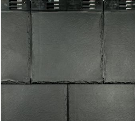
Always lay tiles in half bond.
